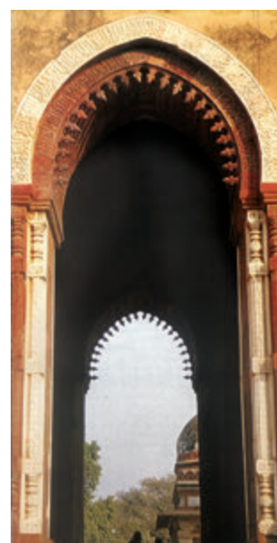
Fig. 5b True arch; detail from the Alai Darwaza (early fourteenth century). Quwat al-Islam mosque, Delhi.
