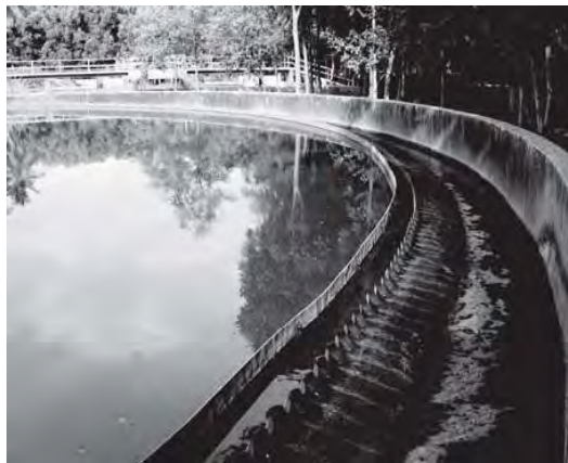
Fig.18.5 : Water clarifier
